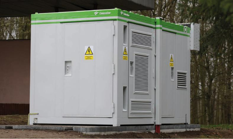
This station is installed in areas where the OCS does not meet the energy requirements for trolleybuses. Typically, these areas are located some way from power substations as the long-distance resistance of the wires causes a voltage drop. The station is installed in cases where the catenary is powered by only one converter station, typically during reconstruction. The buffer station can provide good compensation for a lack of voltage in the system.
