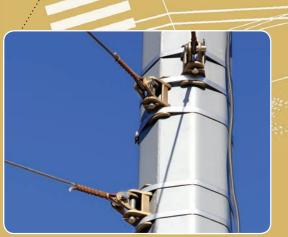
Cross-wire suspensions are fixed to the poles by the various hinge types.
