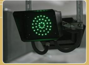
Green color of lamp informs operators about no-voltage status and about the possibility of maintenance close to OCL.
