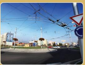
For roundabout solution is suitable use of double switch point controlled by VETRA system with fully automatic operation.
