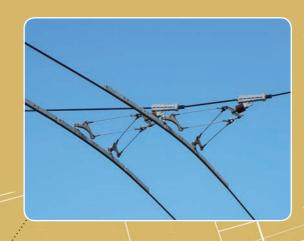
Supporting net made from KEVLAR synthetic ropes decline undesirable noise which is characteristic for vehicle's moving.
