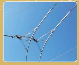
The curve clamps are designed for high-speed operation of vehicles
