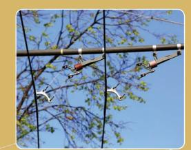
Curve clamps fixed on GRP cantilever
